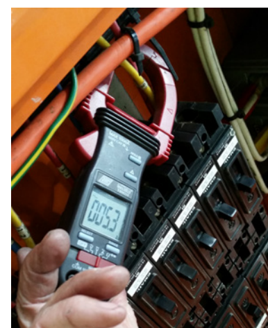
Lighting circuit load testing
